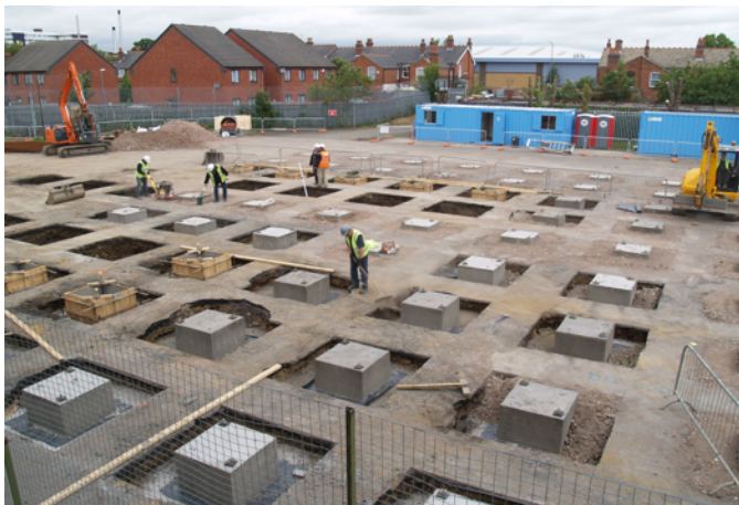
Work starts to prepare the site for the temporary school
