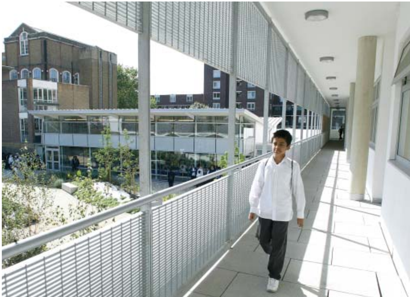
The open walkway of the new modern-languages classroom block with the original Victorian school building (not currently used by the school) and the extended dining room in the background
