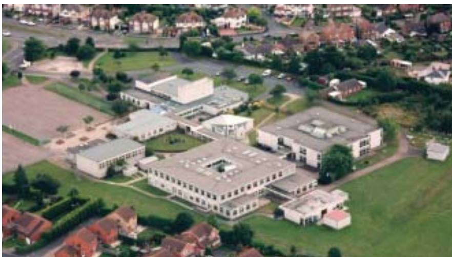
Aerial view of school prior to building work
