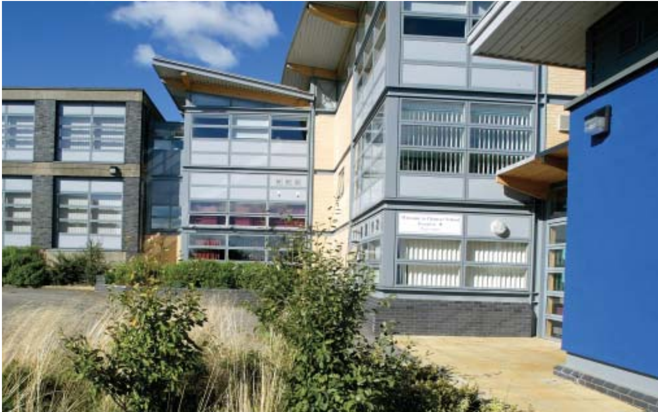
Landscaped central quadrangle, with new science, art and technology link block between remodelled music/drama block on the far right (with new main entrance in between) and refurbished teaching wing to the left
