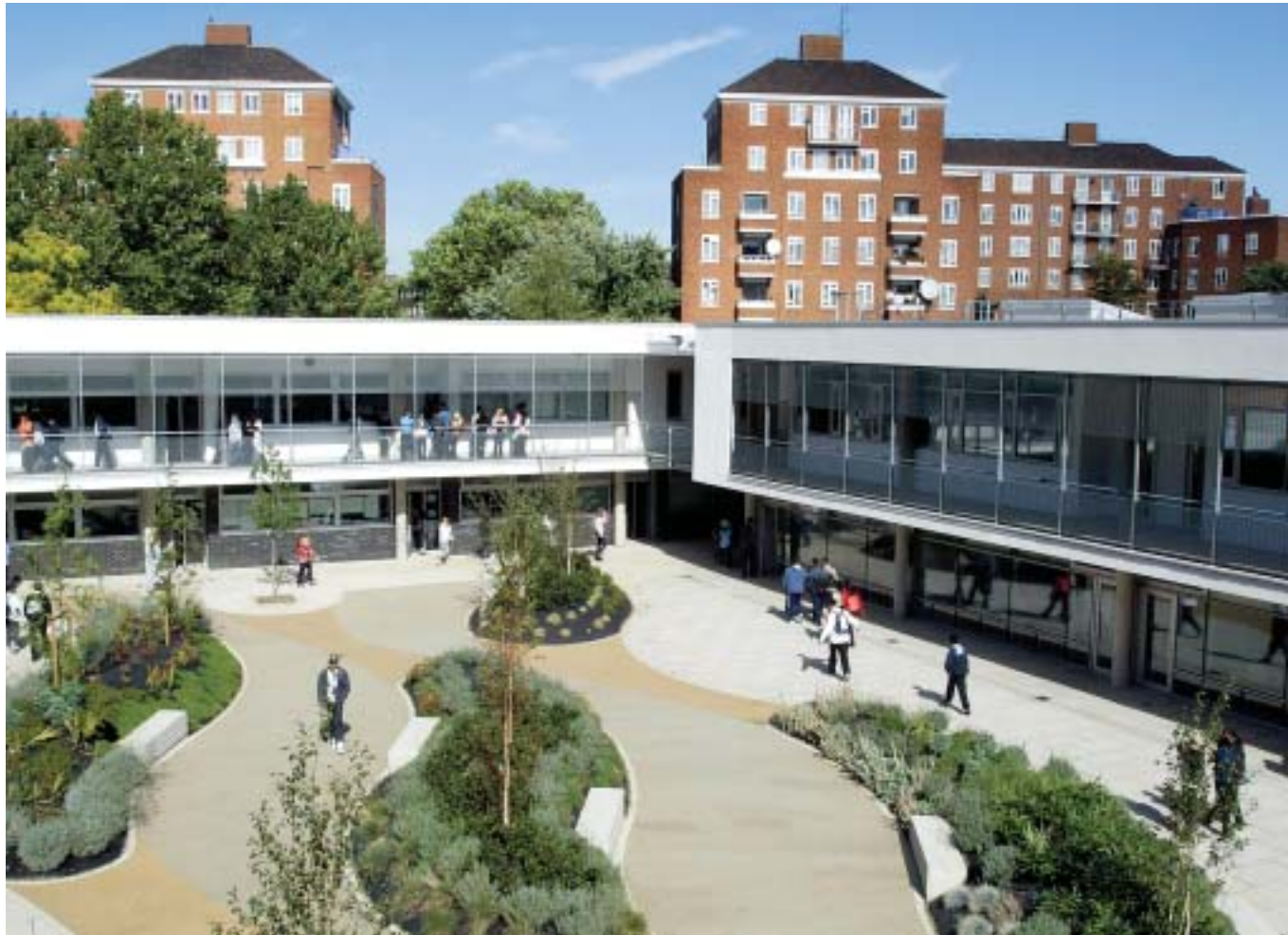
Two new classroom blocks, one replacing poor quality workshops enclose a newly landscaped courtyard, once occupied by shabby and unsuitable buildings
