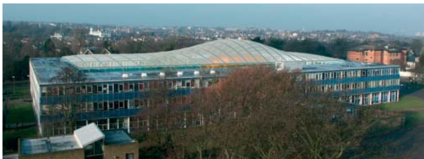
The ETFE roof from above
