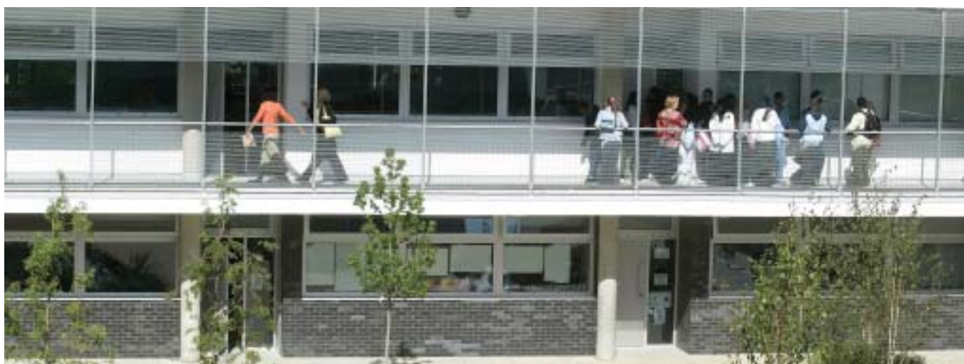
Below: Metal grilles provide shading to the first floor walkway and first and ground floor classrooms in the new modern-languages block
