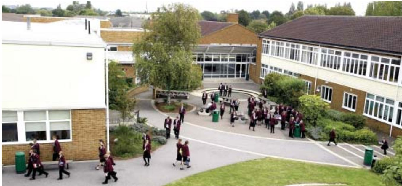
Phase 1 included a new social area with access to an amphitheatre in the courtyard. Phase 2 added practical rooms in the new rear block (left) and phase 3 remodelled the existing two-storey block (right)
