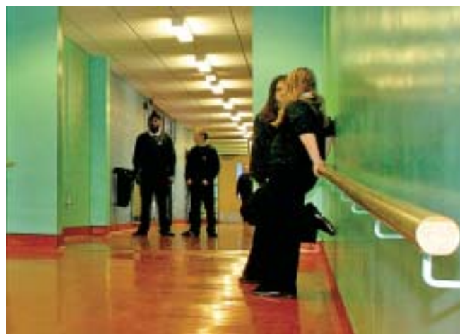
The corridor connecting the new link block to the refurbished teaching wing is ramped to improve disabled access. Paint colours and flooring were carried through to existing areas to unify the scheme
