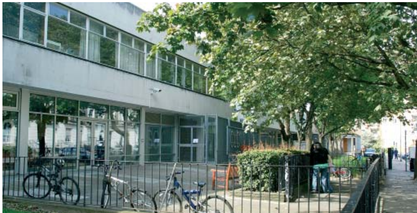
The 1960s main teaching block with cantilevered upper floor. The scale and strong articulation of this elevation have been continued in the new buildings
