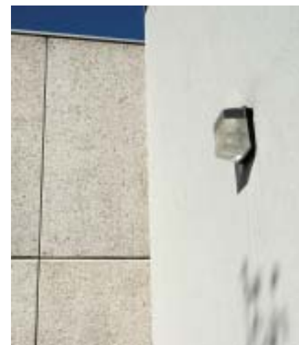
The render used for the new block was chosen to soften the concrete panels on existing buildings
