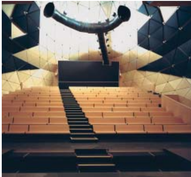
The auditorium interior showing the practical art work which acts as a ventilation duct and lighting boom
