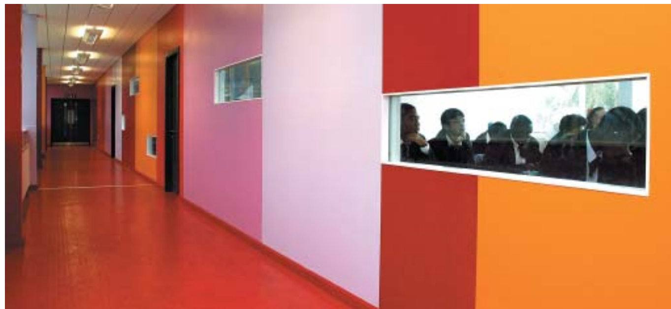
Existing corridors have been transformed by improved lighting, views into classroom activities and a lively colour scheme
