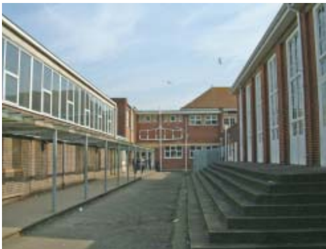
A long thin courtyard along the back of the hall and old gymnasium which subsequently formed the dining room did little to enhance the site
