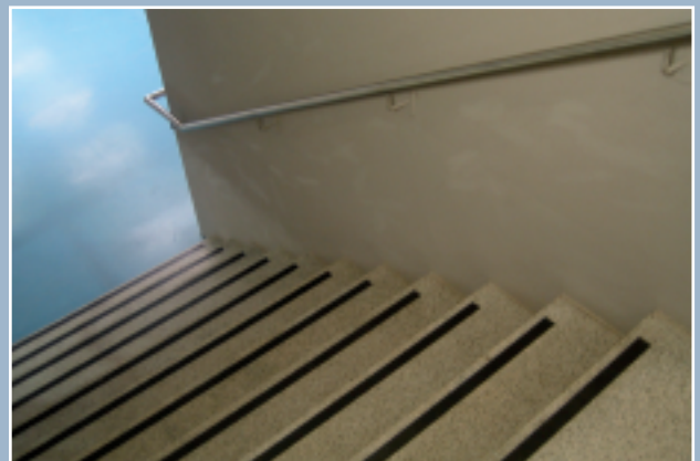
▲ Above carborundum strips set into pre-cast terrazzo treads on pre-cast concrete stair and an in-situ concrete central wall between flights instead of a balustrade
