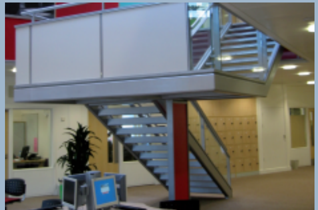
▲ Above free standing stair in learning area
