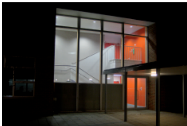
▲ Above Type A stair with glazing assists wayfinding
