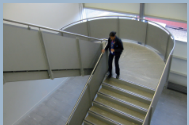
▲ Above free standing steel stair with vinyl sheet floor finish to treads and landings in stairwell
