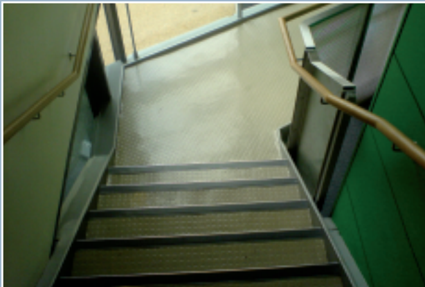
▲ Above steel staircase with studded rubber sheet finish, timber handrails and metal balustrade
