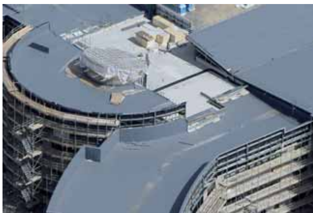
▲ Above continuously supported roof covering
