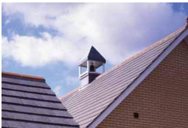
▲ Above discontinuously supported roof covering
