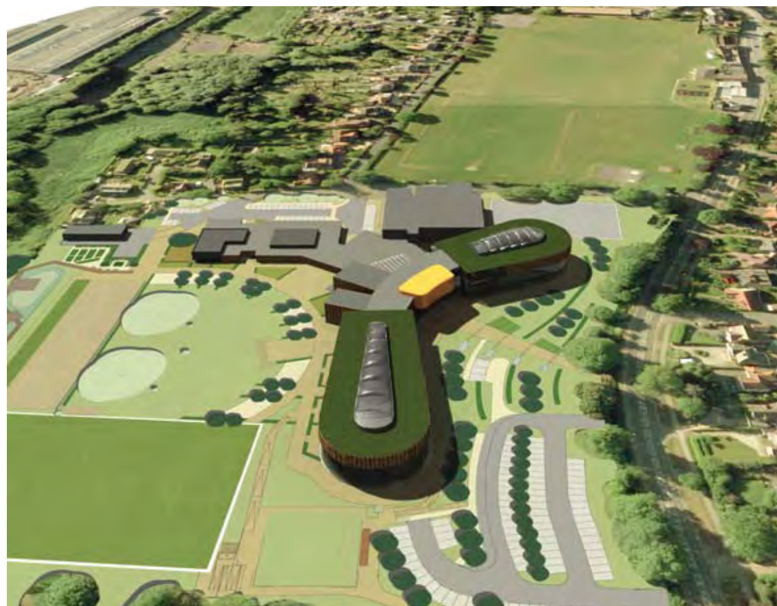
This aerial view of the site shows science accommodation in the foreground, with a large roof light running along its spine.
