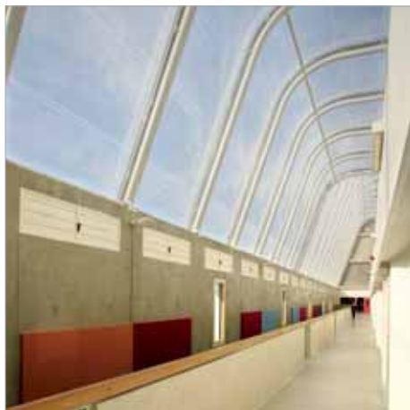
▲ Above Circulation spaces at the Academy of St Francis of Assisi support natural ventilation and good daylight.
