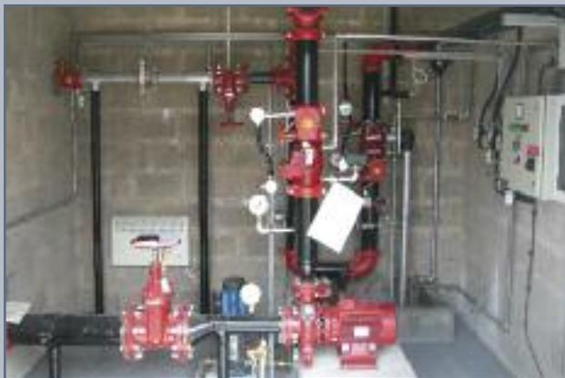
Photograph showing the electric pump and valve set inside the pump house
