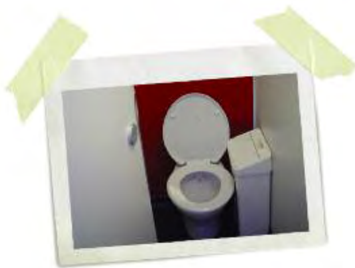
▲ Above allow enough space for sanitary disposal bins, unlike shown here
