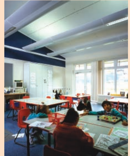
Typical classroom showing monopitch sloping roof, with concrete surface exposed internally, and suspended light fittings with acoustically absorbent casings
