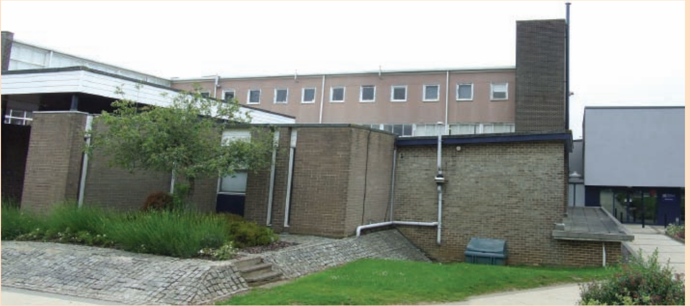
Writlington School existing building
