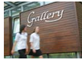
Above: using the delivery entrance, and exterior of the Michael Heseltine Gallery, Chenderit School
